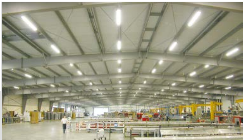
Large free span for optimum utilisation of the available floor - Flexibility of use: to extend-, or to change the use of the building or to incorporate new installation
